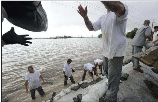
Prisoners from Charleston build an emergency levee on April 27.
